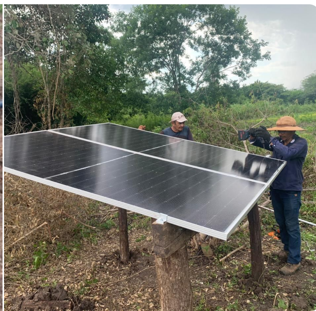
Adaptation strategy in the Pantanal Model Landscape : use of solar panels to reduce electricity costs for pumping water from wells
