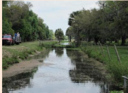
Image 2. Image of stepped riser board system
