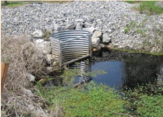
Image 1. Image of culvert and riser board
